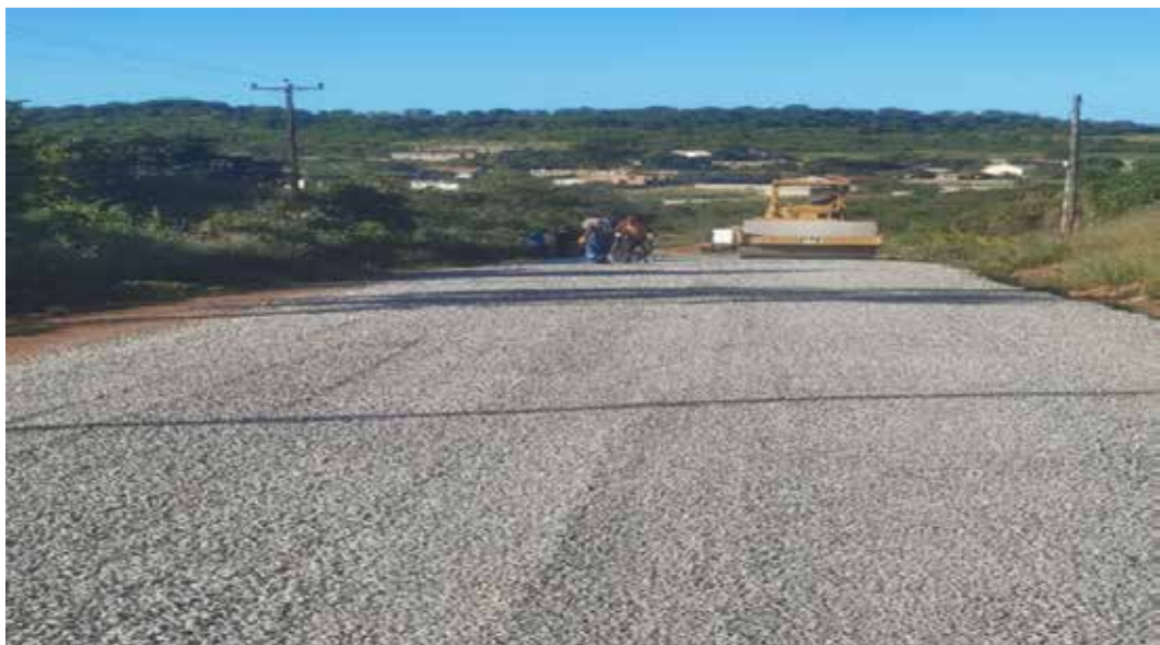
Gwanda Municipality, Jacaranda Road construction
