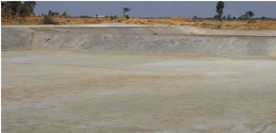
Mvurwi Town Sewer Ponds
