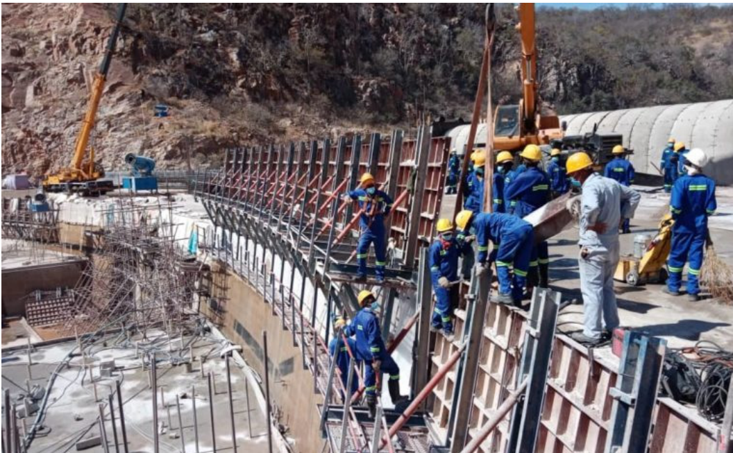
Construction of the Kunzwi Dam
