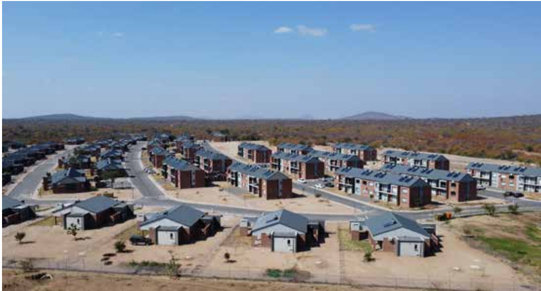
Beitbridge Border Housing. Source: Thembani Media
