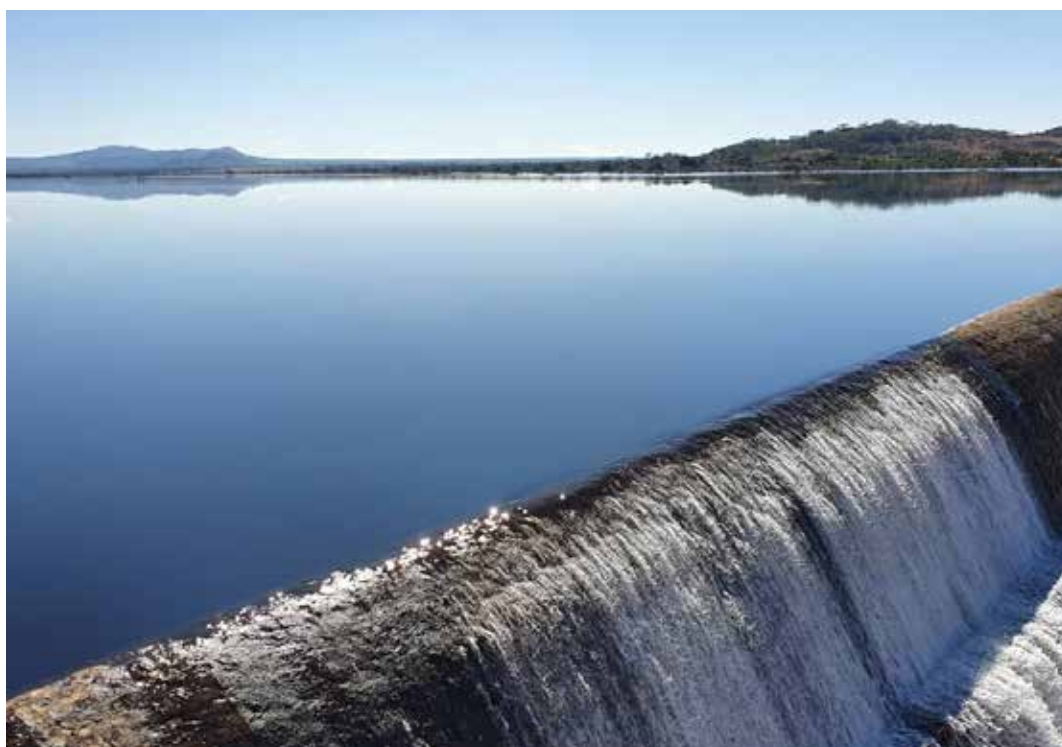
Muchekeranwa Dam in Marondera
