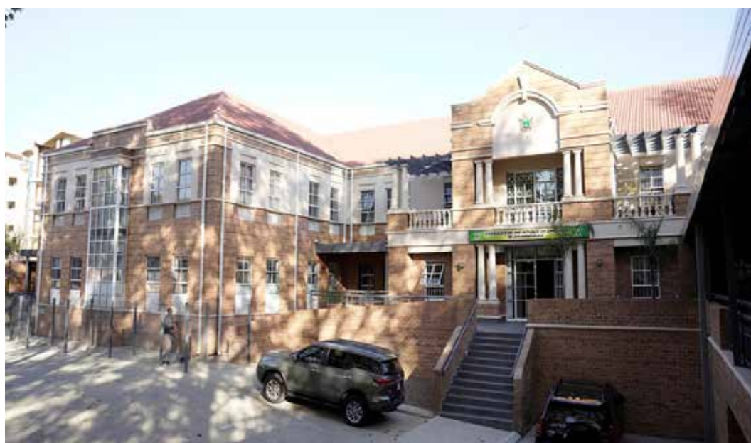
Refurbished Johannesburg Consulate
