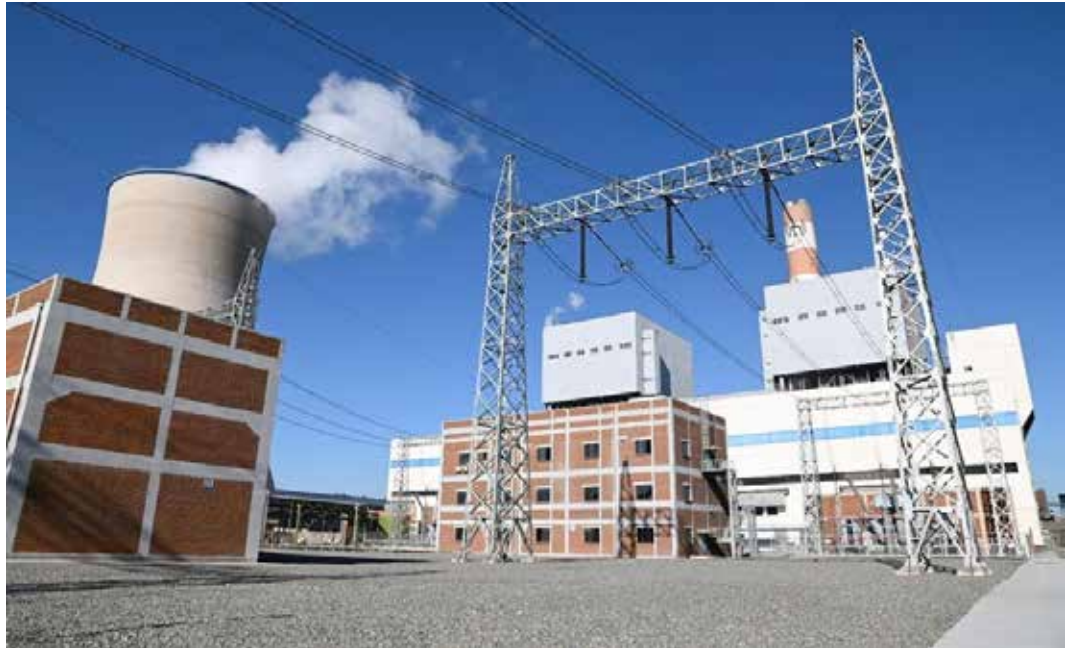
Hwange 7 & 8 Thermal Power Station
