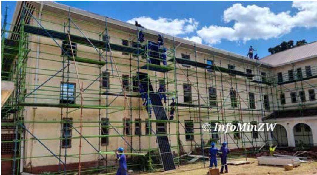
Rehabilitation of the Parirenyatwa Group of Hospitals
